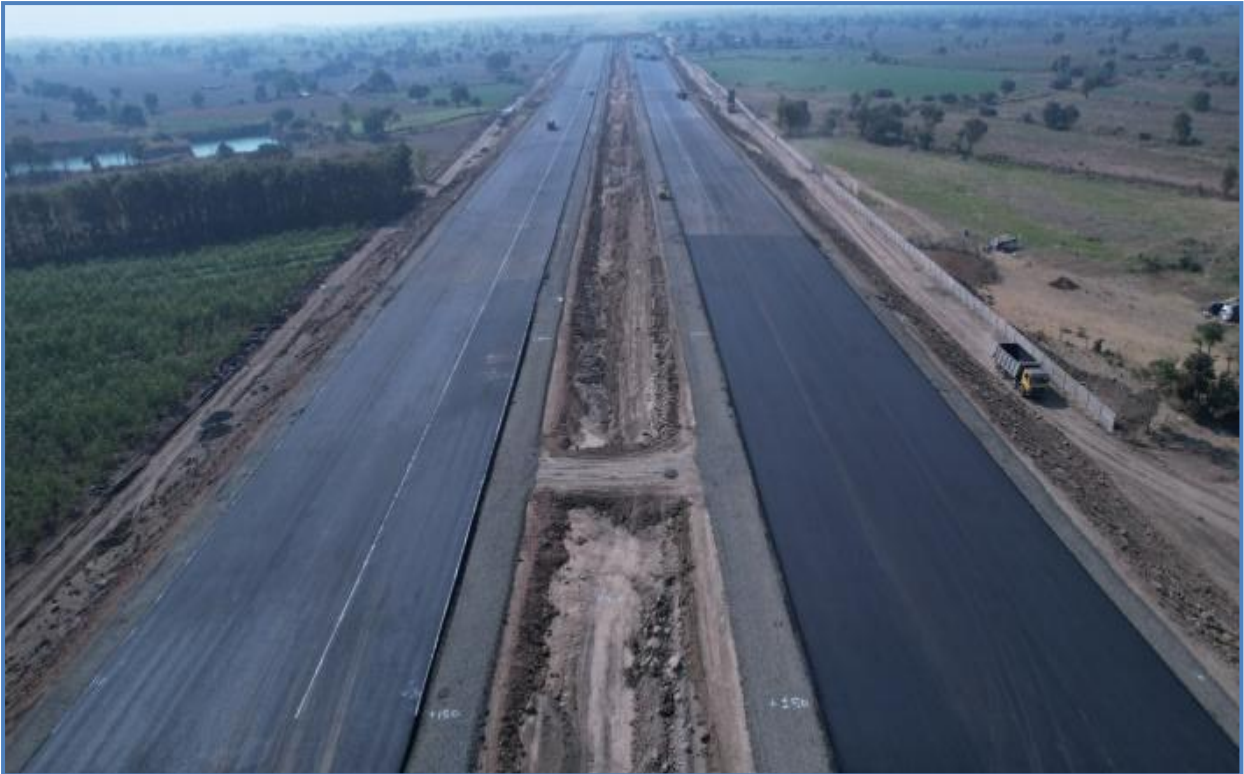
DBM Work In Progress at ch. 362+150 to 362+890
