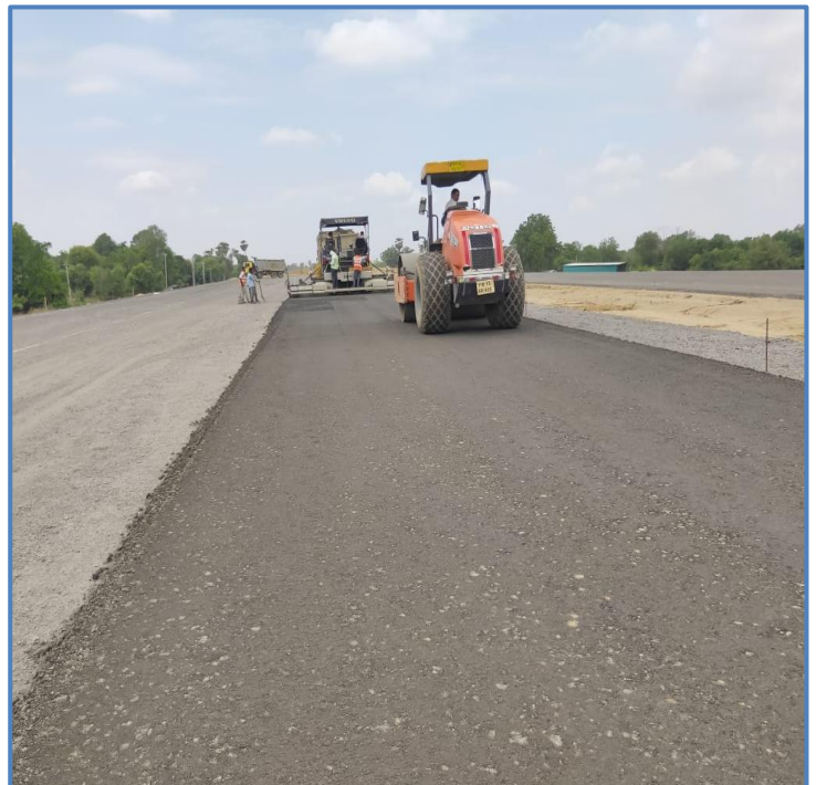
DBM Work In Progress at ch. 362+150 to 362+890
