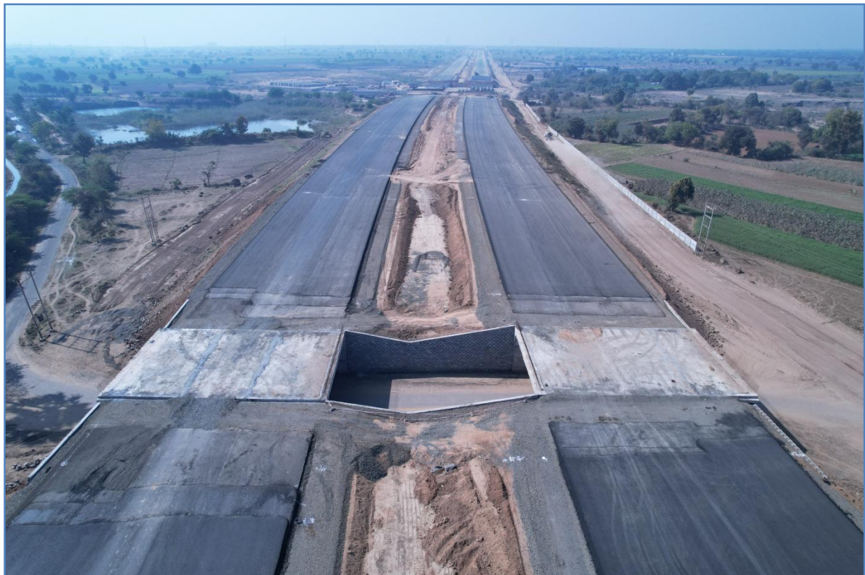
DBM Top Laying at chainage – 359+485 (LVUP Approaches)
