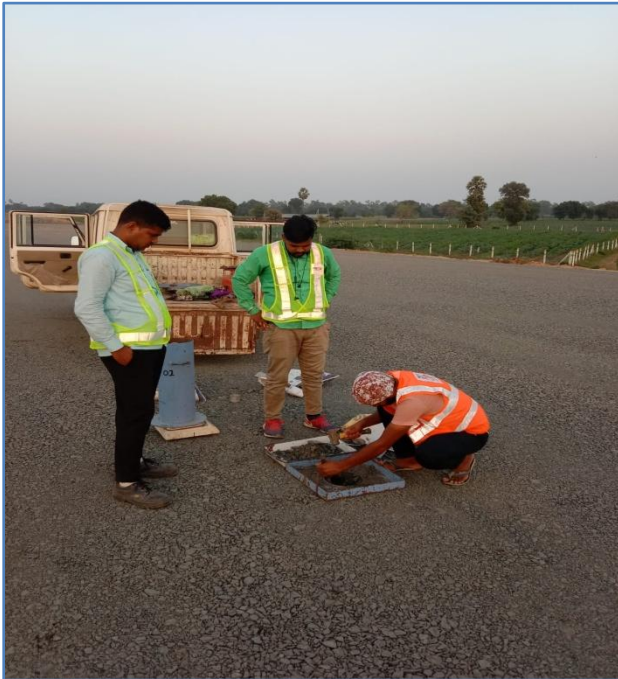
FDD checking at Ch. 351+150 GSB Top
